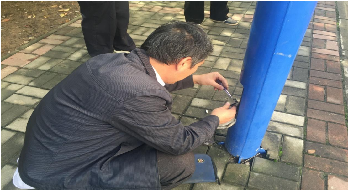
长安校区栾林路检修路灯更换路灯电熔
