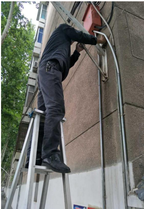
雁塔校区检修变压器箱
