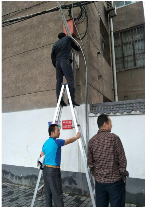
雁塔校区检修变压器箱
